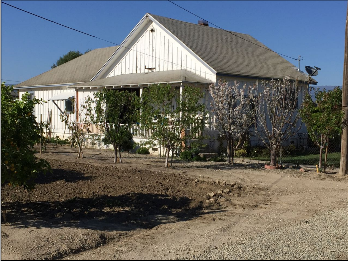
Photo 9. Residence, western and southern elevations. [3-31-17]
