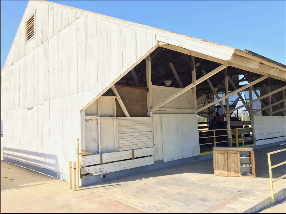
Photo 13. Equipment Shed, southern and eastern elevations. [3-31-17]
