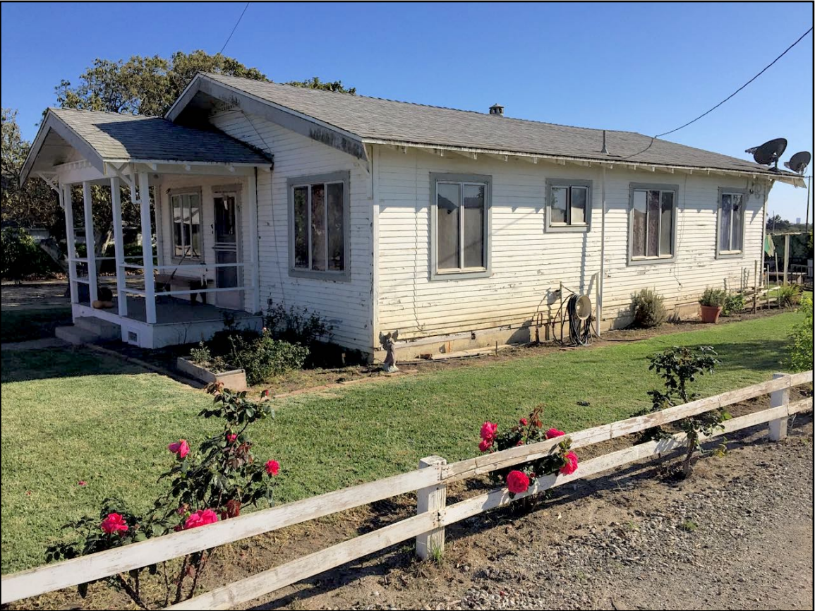
Photo 6. Residence, northern and eastern elevations. [3-31-17]
