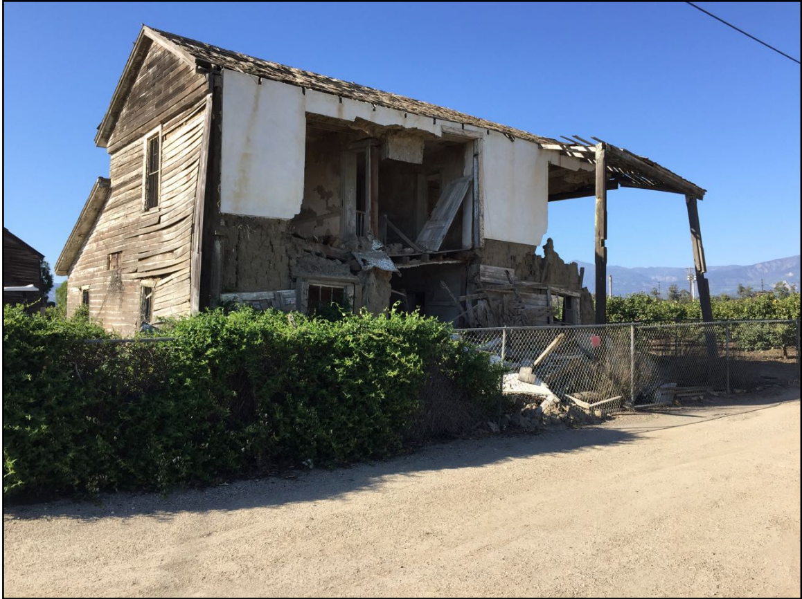
Photo 1. More-Edwards Adobe, southern and western elevations. [3-31-17]
