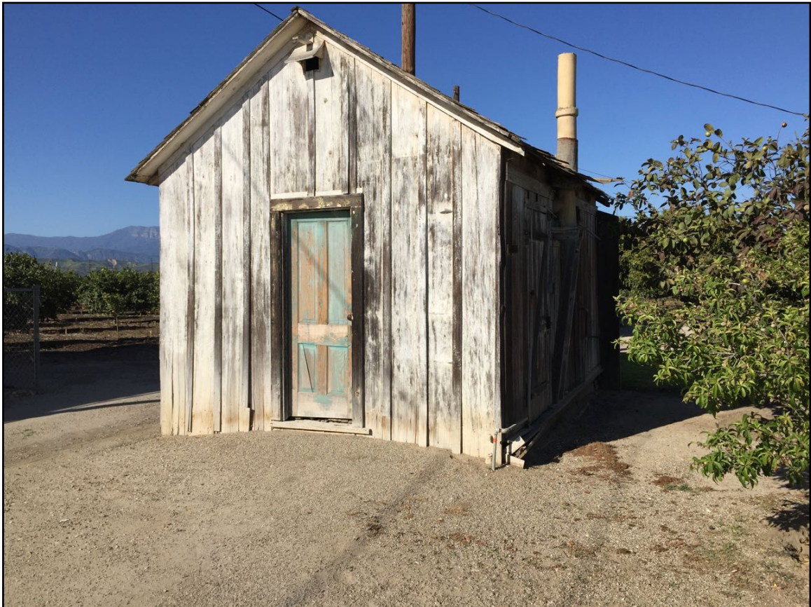
Photo 4. Office Building, western elevation. [3-31-17]
