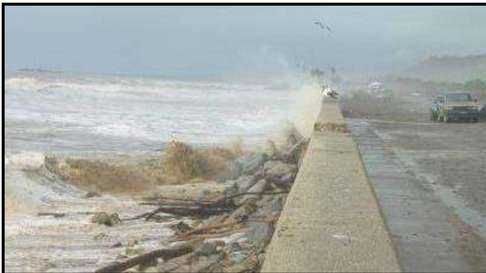
**Photo 2-5. This seawall is a form of coastal armoring that is located along the Rincon Parkway. Photo taken during a large wave event (source: D. Revell).**
