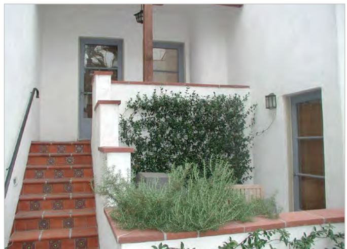
Image 6.16. A plastered masonry wall capped with terracotta tiles.
