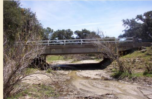
Bridge for Canada Verde Creek and the PCT under SR-79.
