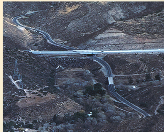
Agua Dulce Canyon vehicle underpass, with drainage culvert for stream visible to the left of the underpass.
