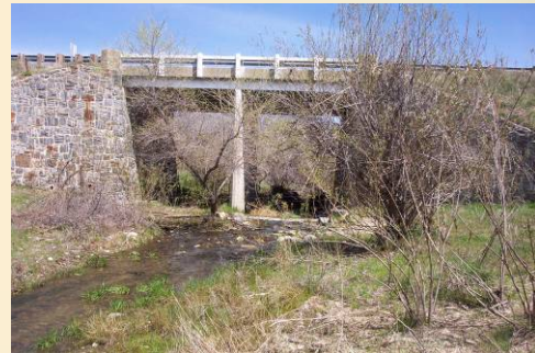
Bridge for Santa Ysabel Creek on SR-79.
