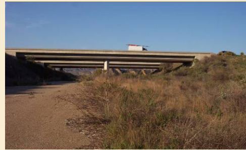
Looking toward the Santa Susanas through the bridge at Alamos Canyon.
