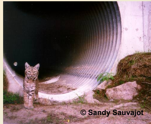
Pipe culvert north of Tierra Rejada; typical of most structures on SR-23.
