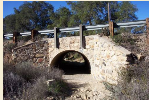
Kolb Creek bridge on the SR-79.
