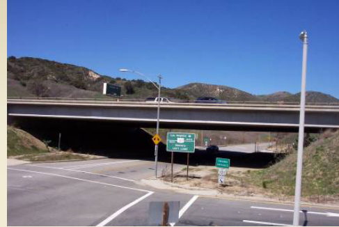
Looking toward the Simi Hills through the Liberty Canyon underpass.
