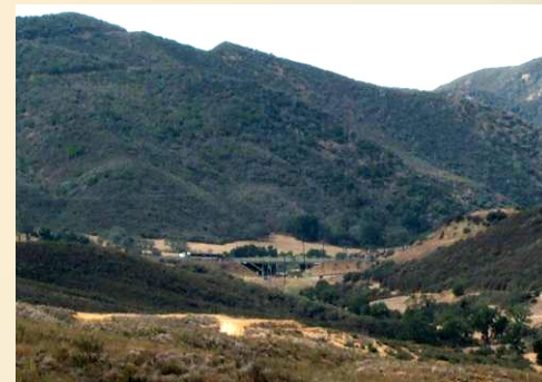
Canton Canyon with Templin Highway underpass at the center of the photo.
