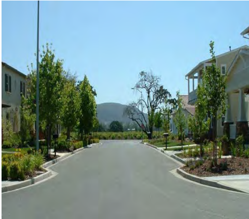
Bulb-outs, as seen in the foreground, slow traffic, and create safer pedestrian crossings.
