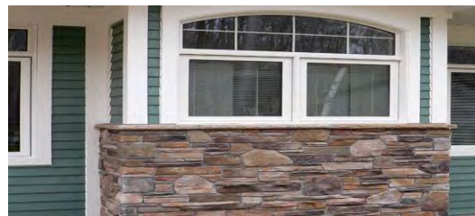
The base of buildings should be comprised of heavier materials and/or colors.
