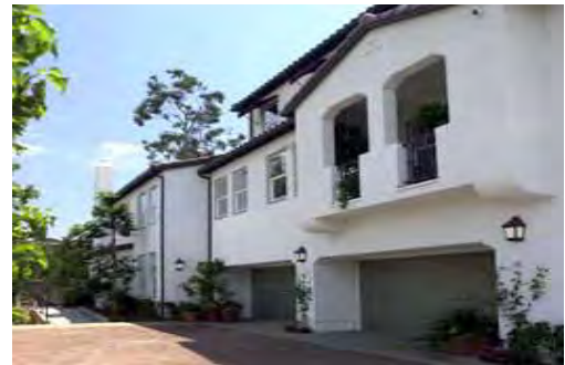
Attached garages are preferred in multi-family developments.
