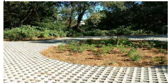
Grass pavers allow infiltration of stormwater while providing a load-bearing surface. This picture shows the project in the final stages of completion. The voids between the concrete lattice structure should be filled with a loamy material to allow for sufficient infiltration rates.
