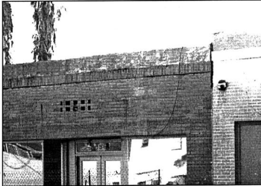
A concrete parapet rests atop a soldier course of brick on a shop building in Piru's unique Commercial Town Center.
