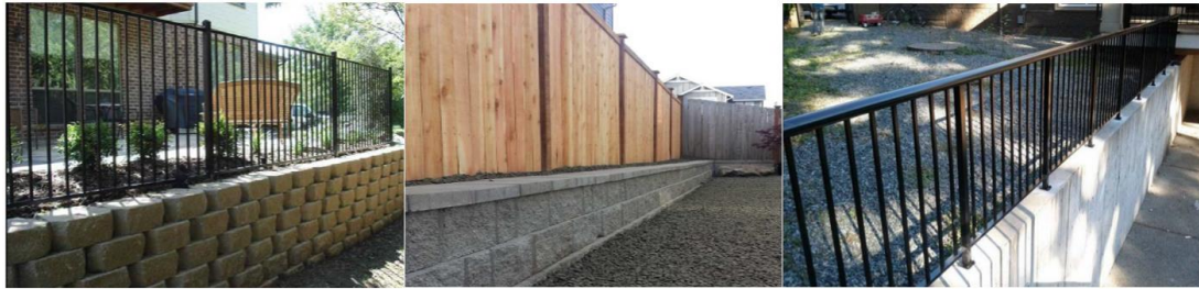
Examples of Fences on top of Retaining Walls
