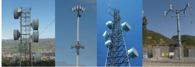
Examples of Non-Stealth Wireless Communication Facilities (ADD. ORD. 4470 – 3/24/15)
