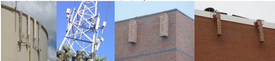
Examples of Flush Mounted Wireless Communication Facilities (ADD. ORD. 4470 – 3/24/15)
