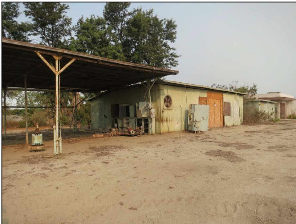
Figure 15. View of the Maintenance Shop, looking northwest.
