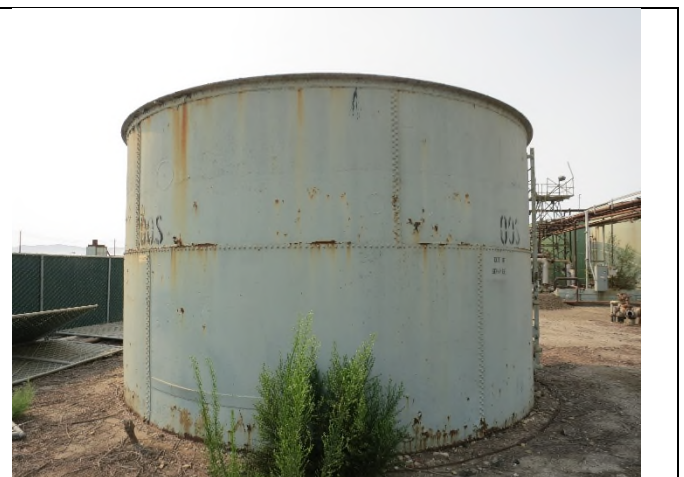
Image 6. Tank 501 looking south.
