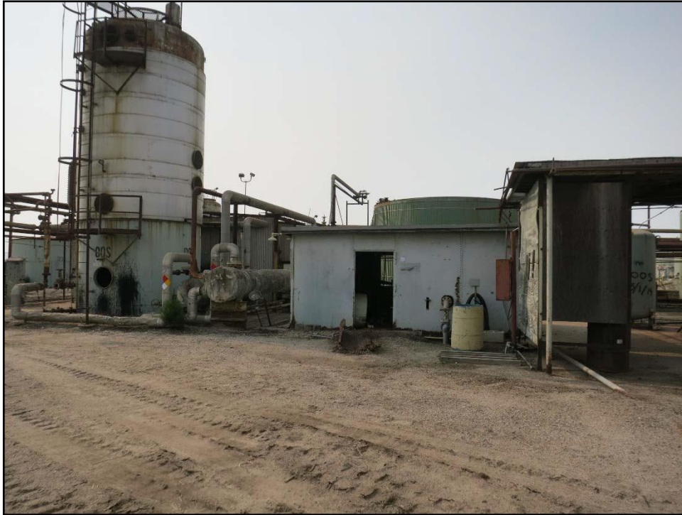
Figure 22. Shed in Chemical Processing area, looking south.
