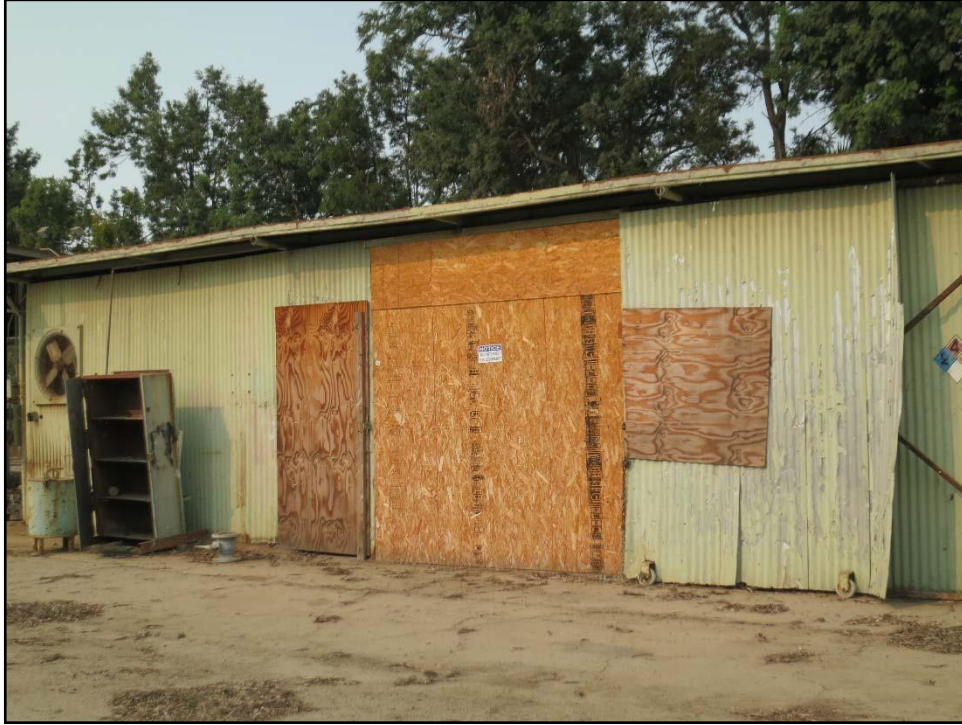
Figure 16. Detail view of primary (east) façade of Maintenance Shop, looking southwest.
