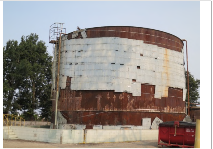
Image 2. Tank 12001 looking west.
