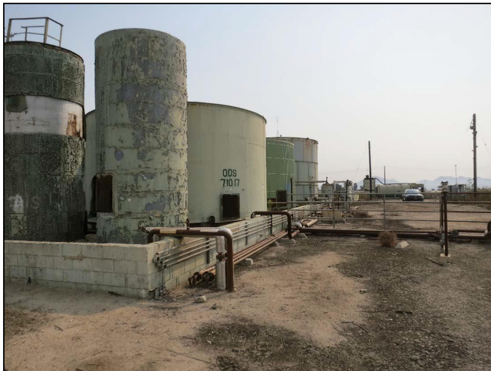
Figure 32. Tanks 2011, 2012 and water tank, looking east.
