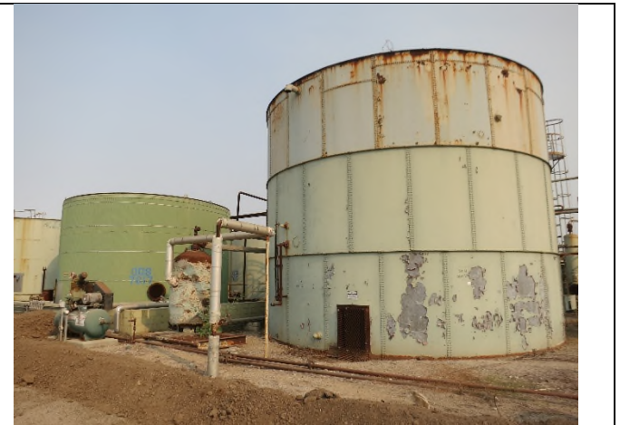
Image 4. View of Water Tank looking northwest
