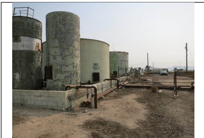
Image 5. View of tanks looking east.
