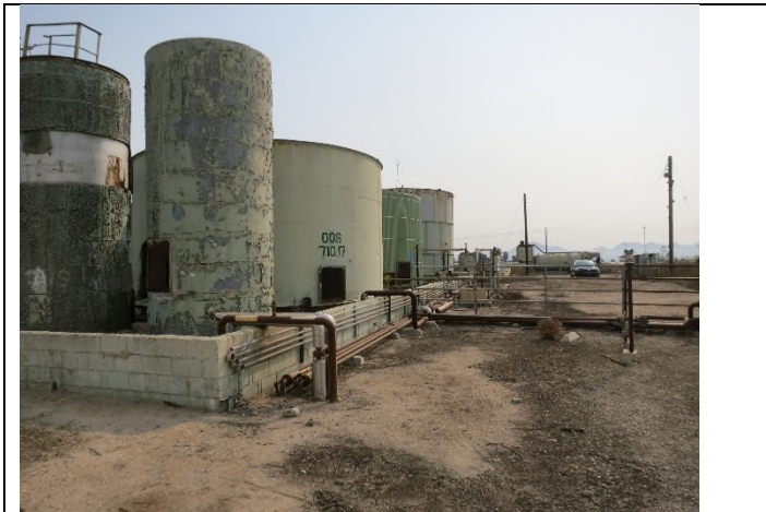
Image 3. Tanks 2011, 2012 and water tank looking east.
