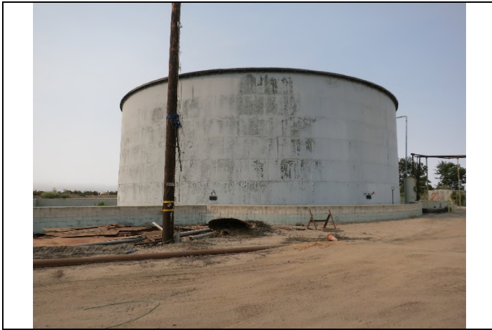
Image 1. Tank 30001 looking south.
