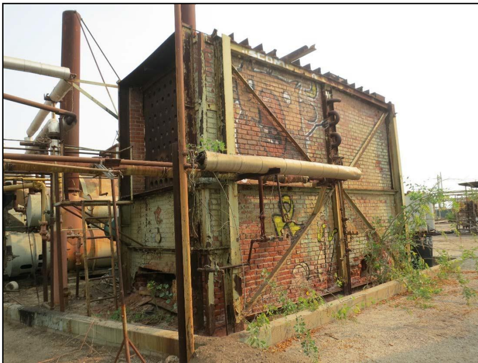
Figure 44. Brick heater, looking northeast.
