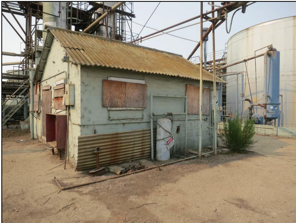
Figure 13. North façade of Control Room, looking southwest.
