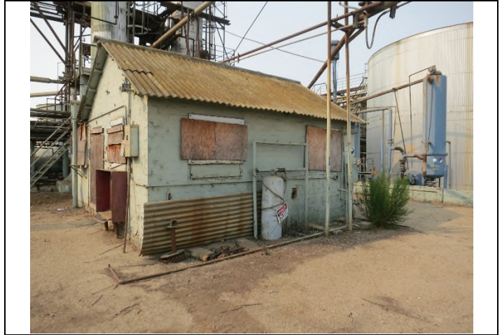
Image 2. North façade of Control Room.
