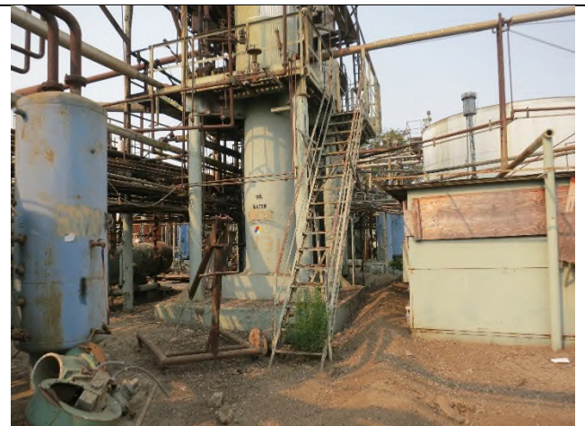
Image 6. Smaller tanks and equipment looking south.
