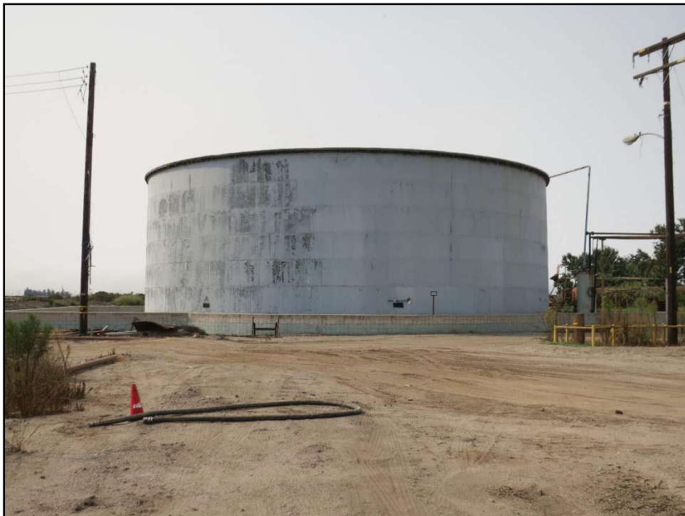
Figure 38. Tank 30001, looking south.
