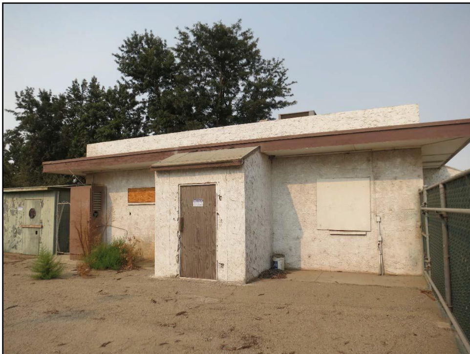
Figure 19. East façade of Lab, looking southwest.
