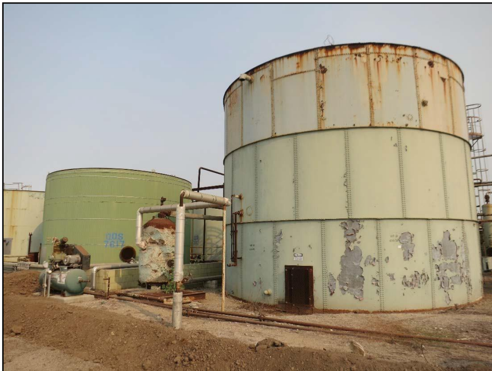
Figure 34. View of Water Tank, looking northwest.
