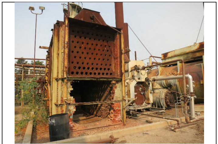
Image 4. Brick heater looking northwest
