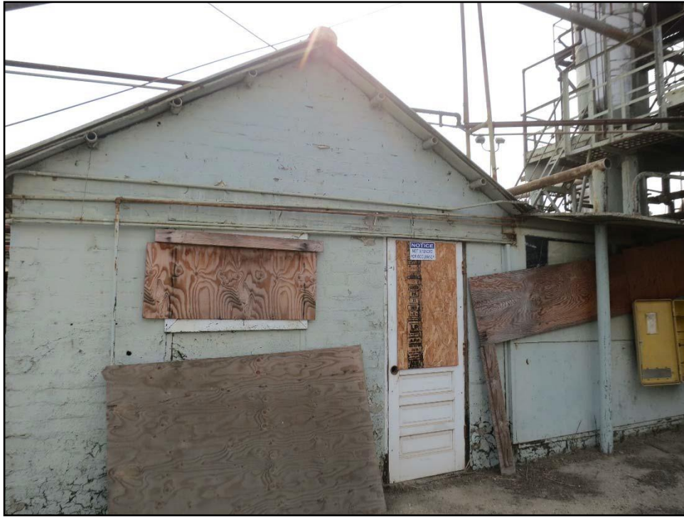
Figure 14. West façade of Control Room, looking southeast.
