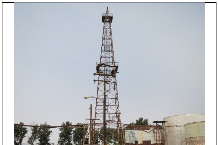
Image 6. View of Derrick looking west.
