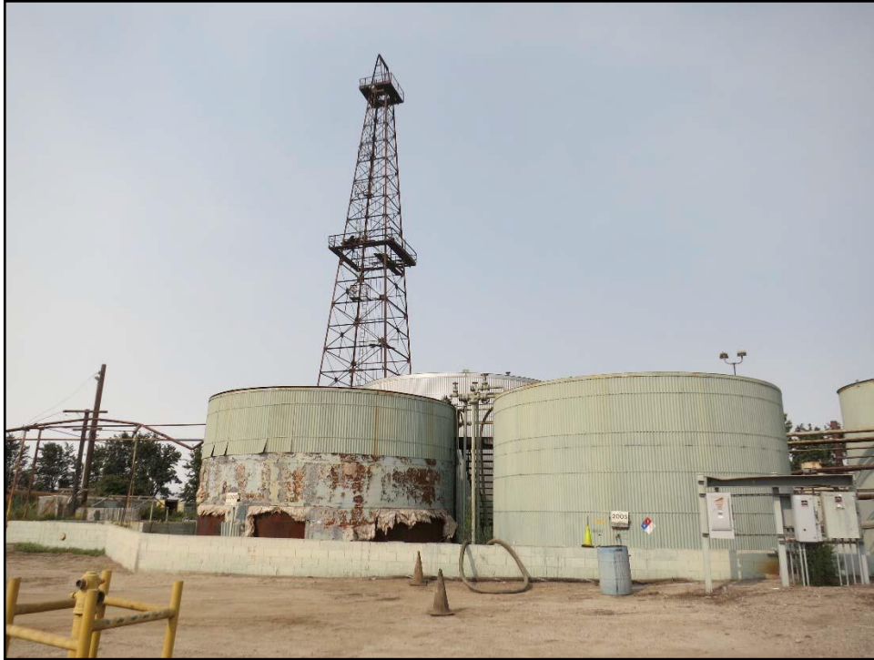
Figure 31. Tanks 2006 (on left) and 2005, looking southwest.
