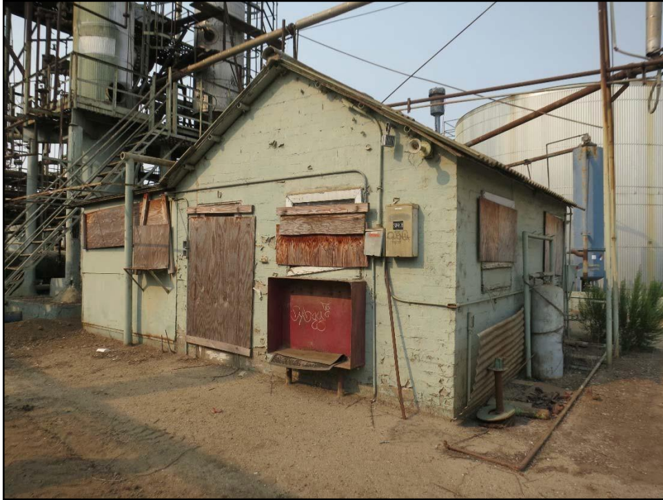
Figure 12. East façade of Control Room and distillation towers, looking southwest.
