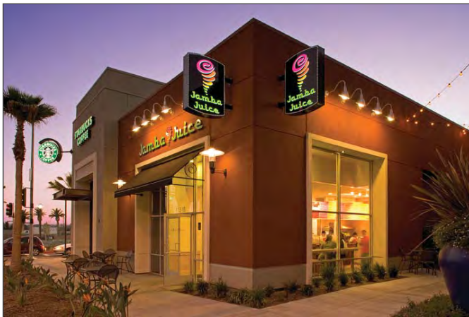
A one-story commercial building with street-facing windows.
