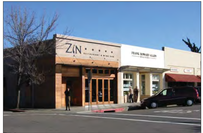
One-story commercial buildings.
