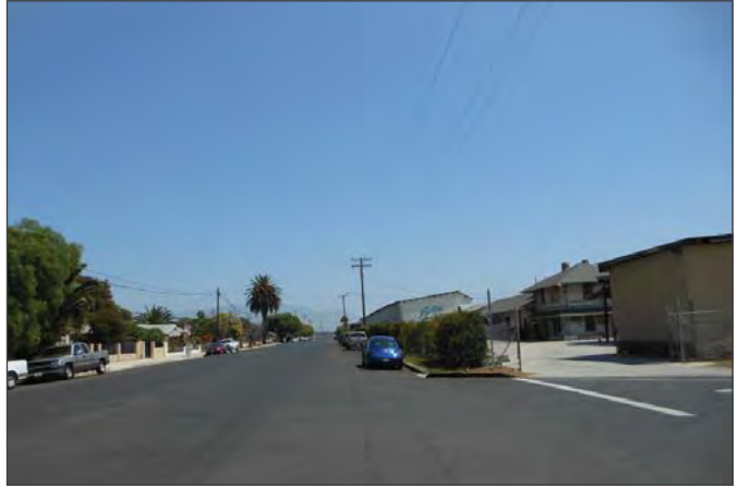
Existing view of Azahar Street at Alelia Avenue looking east with the train depot to the right
