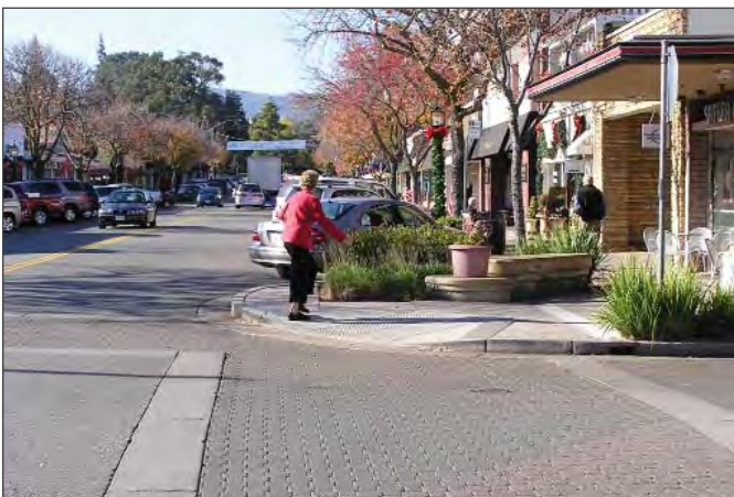
A bulb-out reduces pedestrian crossing distances, slows turning cars down, and provides a place for landscape and street furniture.
