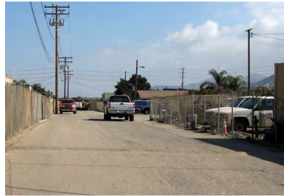
View of Lirio Extension, located close to the end of Lirio Avenue
