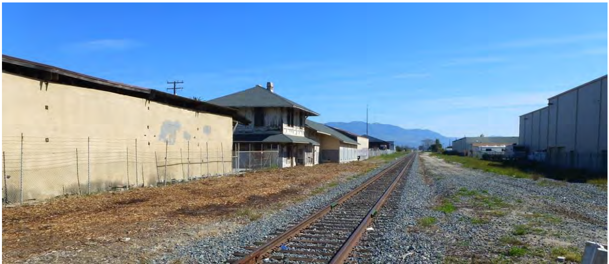
View of railroad right-of-way looking east, with the two-story Depot to the left of the tracks
