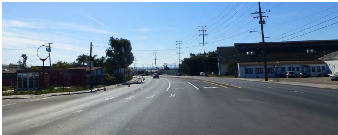
View of SR 118 (Wells Road) at Violeta Street.
