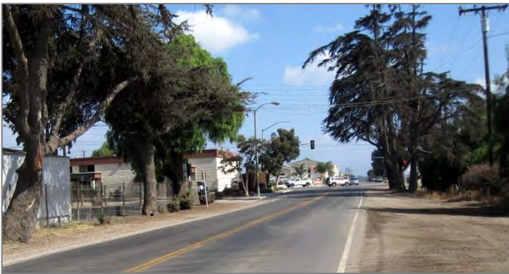
There are no sidewalks present along the entire length of Nardo Street in the west industrial area.
