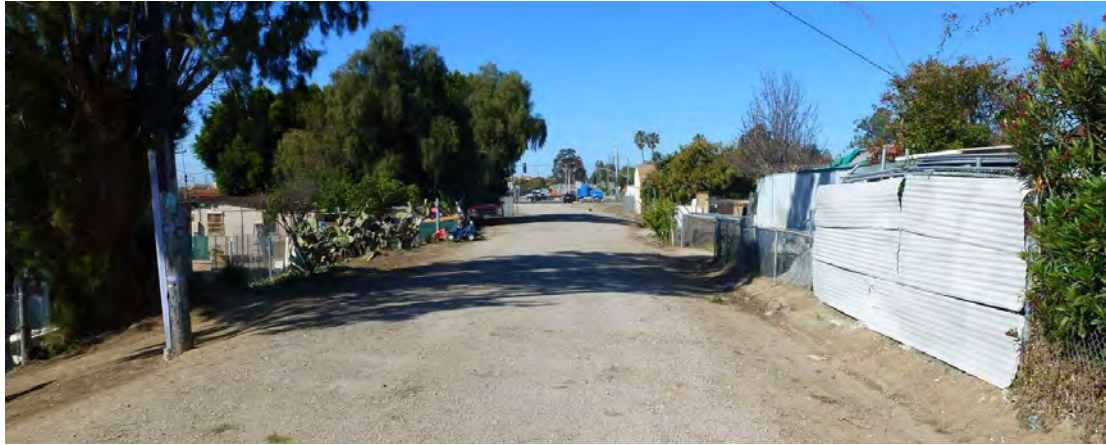
View of buried stormwater drainage pipe that runs along the Telephone Road alignment.
