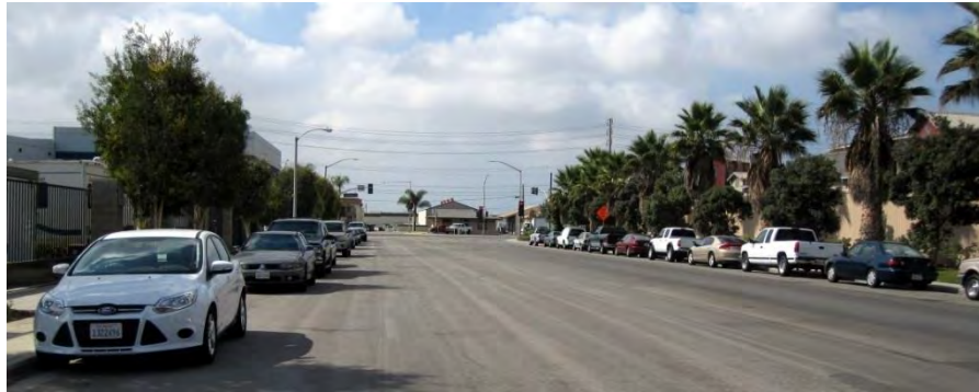
View of County Drive looking west towards Wells Road.
