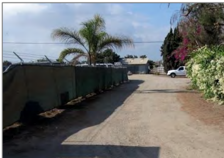
View of the access to Lirio Extension from the private easement.
