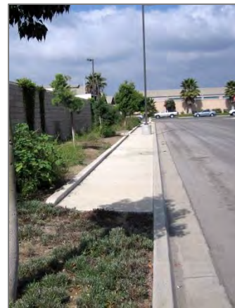
The sidewalk on the west side of Riverbank Drive accessed from County Drive stops abruptly after 200 ft
