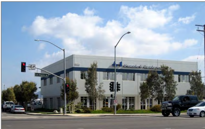
A short length of sidewalk is present at the intersection of County Drive and Los Angeles Avenue.
