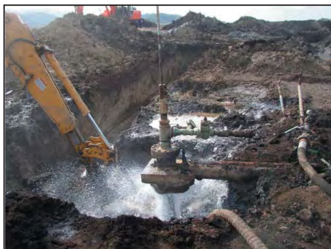
Photo 1. Well "Ojai" 36. During killing operations, vacuum trucks removed water flowing from the well until kill mud could be injected to help secure the well before abandonment operations could begin. Photo by D. Kahler.
