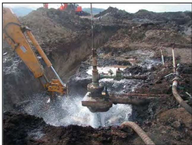
Photo 1. Well "Ojai" 36. During killing operations, vacuum trucks removed water flowing from the well until kill mud could be injected to help secure the well before abandonment operations could begin. Photo by D. Kahler.
