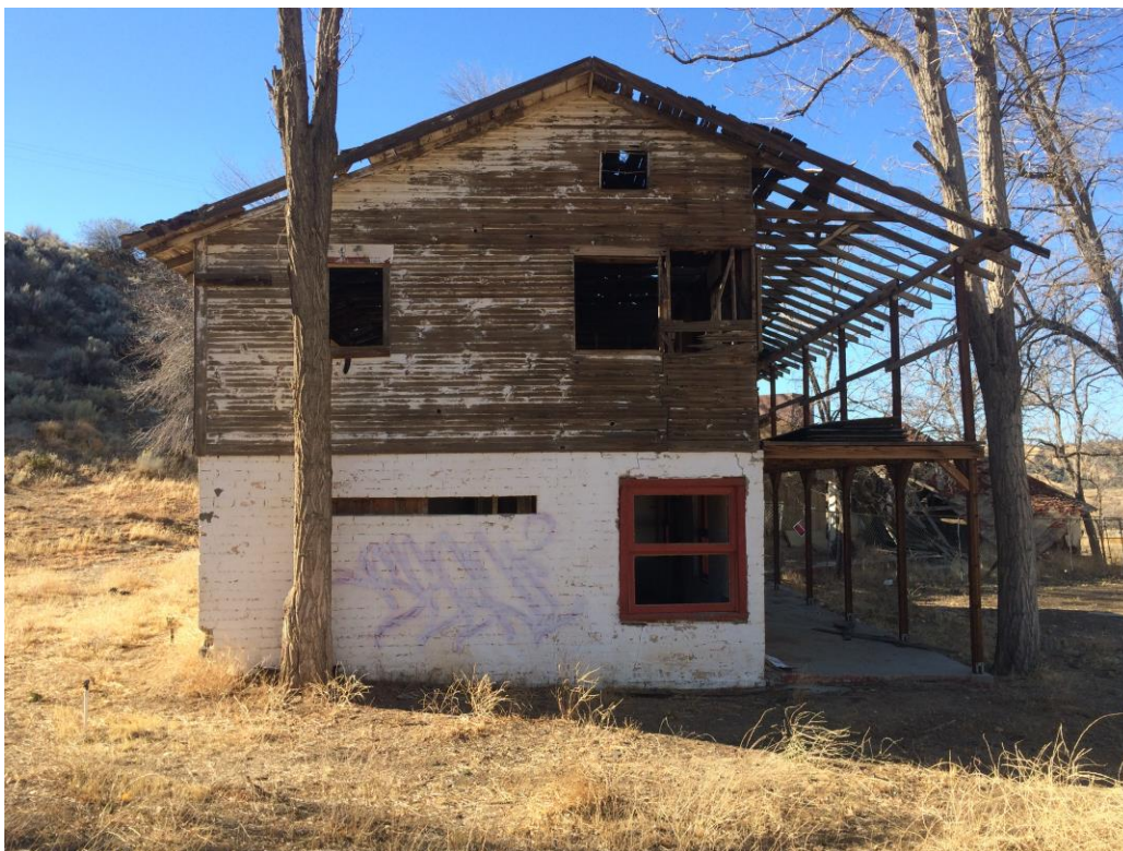
Figure 17. View of south façade of two-story addition looking west.
