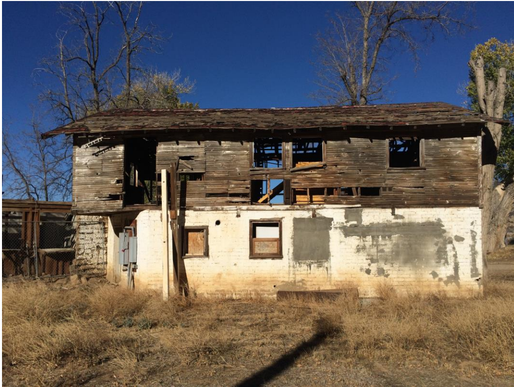
Figure 18. Overview of west façade of two-story addition, view towards the north.
