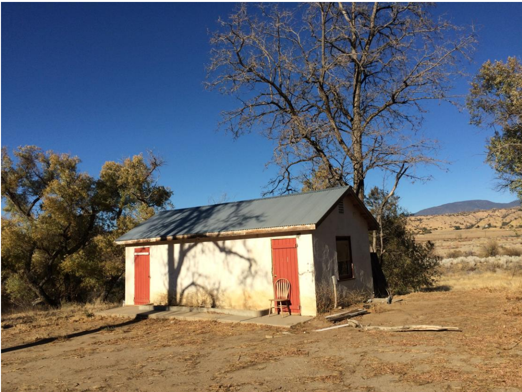
Figure 9. View of cabin on property built 1956, looking northwest.
