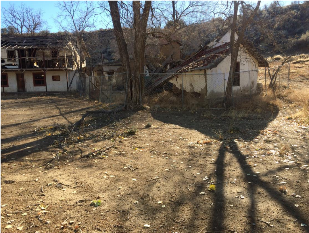
Figure 8. Overview of adobe and addition looking southwest.
