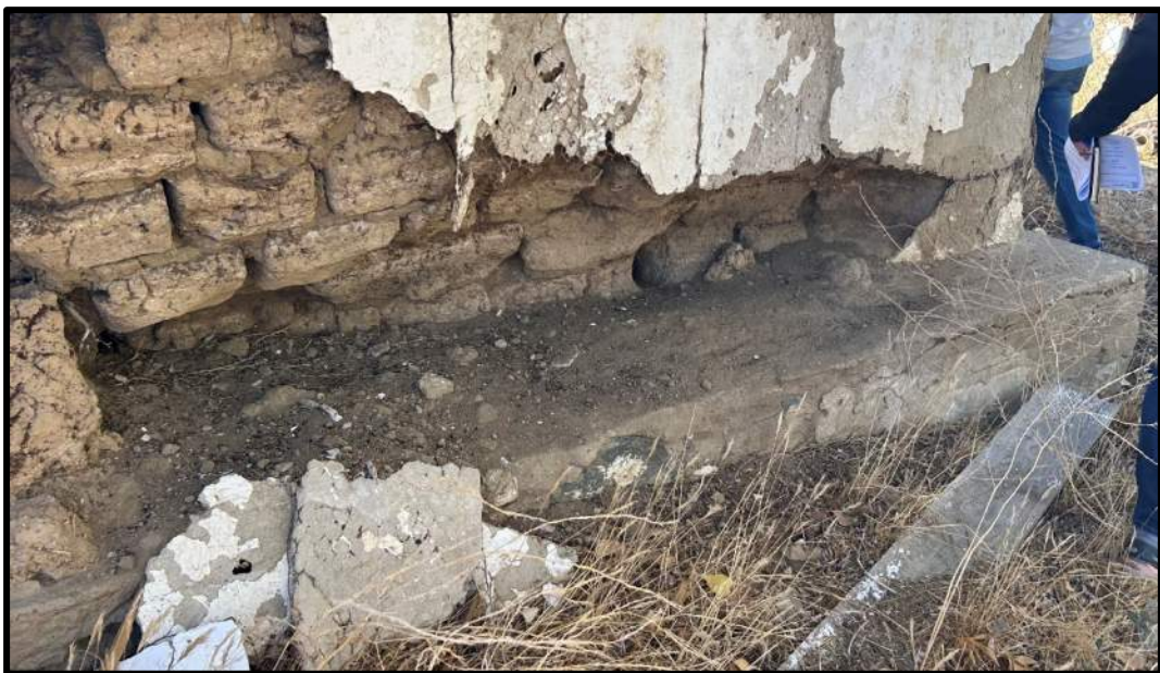
Underpinning Replacing Lower Portion of Adobe Wall
