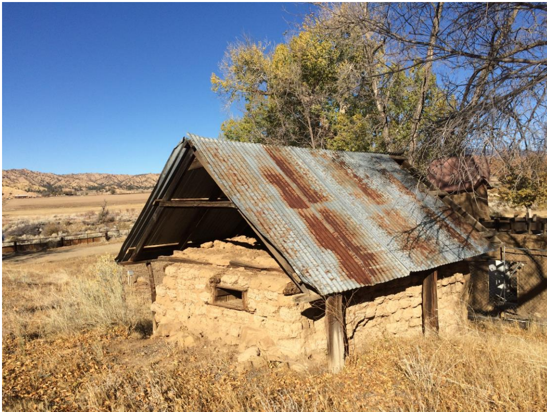
Figure 21. West façade of smokehouse, view to the northeast.
