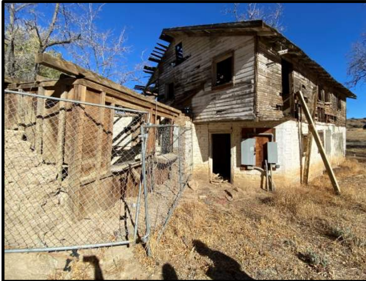
Fence Restricting Access at Adobe Wing (left) of the Building
